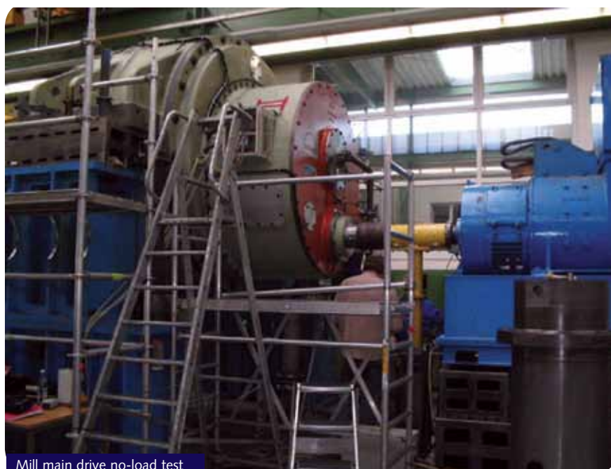
Mill main drive no-load test
